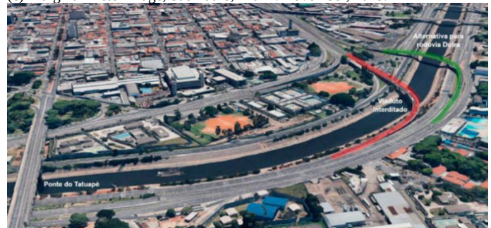
(d) Marginal Tietê / Via Dutra Bridge, São Paulo, Brazil. Interdicted in February, 2019.
