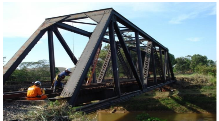
Figure 6. Suaçuí River Bridge - Warren truss with 41m span.
