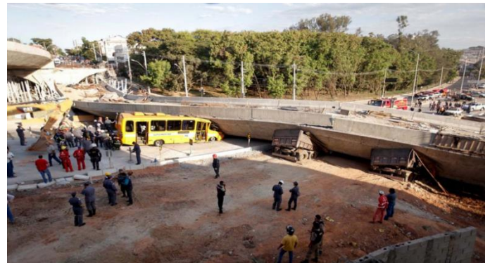
(a) Guararapes Bridge in Belo Horizonte-MG, Brazil. September, 2014.
